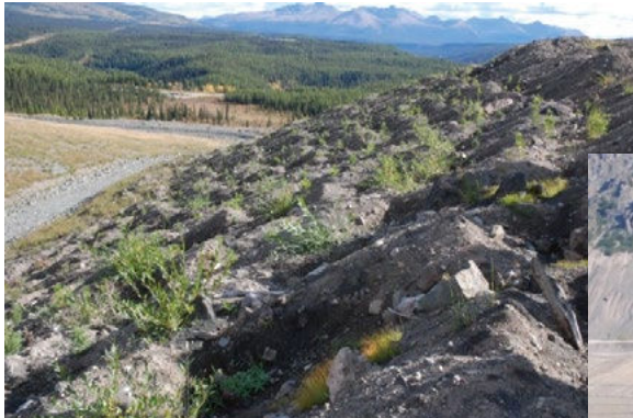
“Re-sloping waste rock dumps and making the surfaces rough and loose creates conditions that promote recovery of these sites.”
